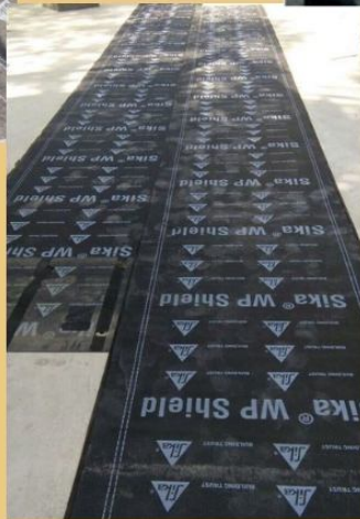
SURFACE TREATMENT ROLL ON MEMBRANE
