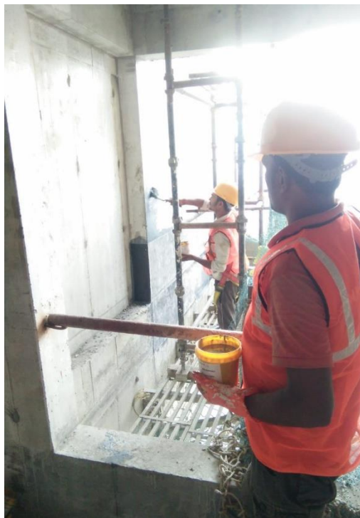
Application of the Carbon Wrap
