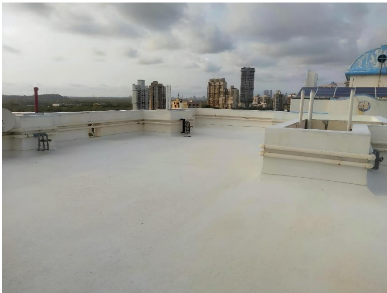
Terrace Waterproofing with Liquid Applied Membrane
