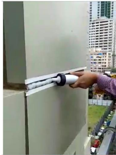
Sealant being filled
